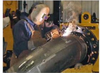
MANUFACTURING OF PUMP SKIDS
